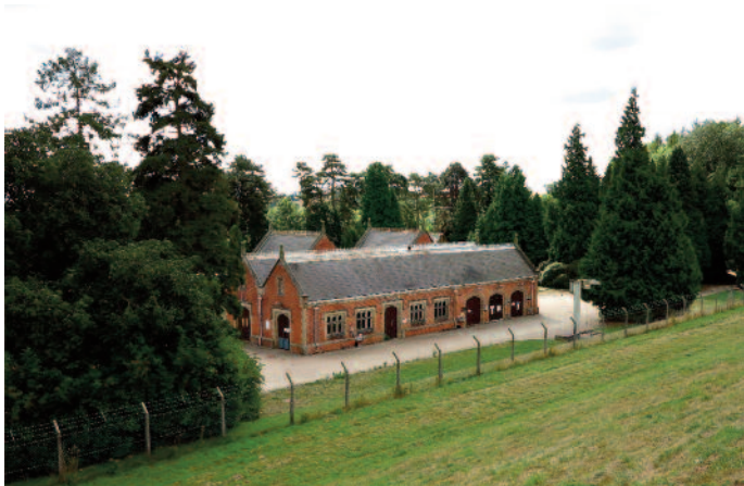
Fig 19 Victorian water treatment works
