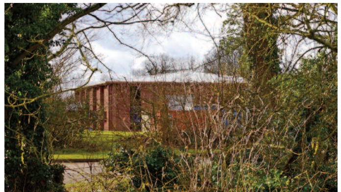
Fig 23 Well screened commercial development Torquemeters factory
