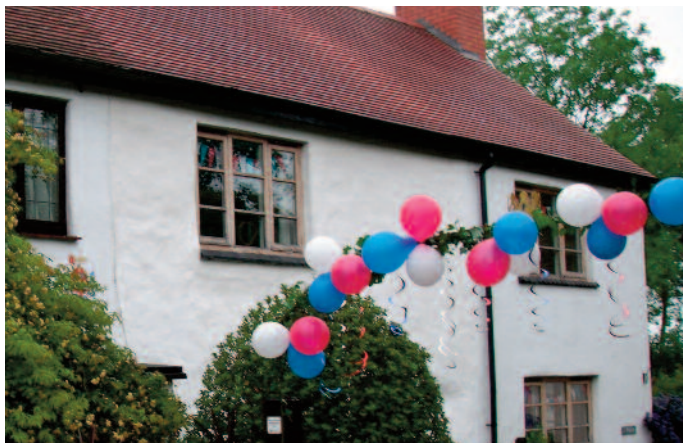
Fig 39 Lime rendered cob cottage
