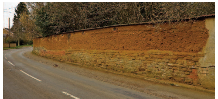
Fig 38 Cob wall with capping on Teeton Road
